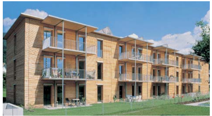
Multifamily house Ölbündt, Dornbirn, Vorarlberg, Austria.
